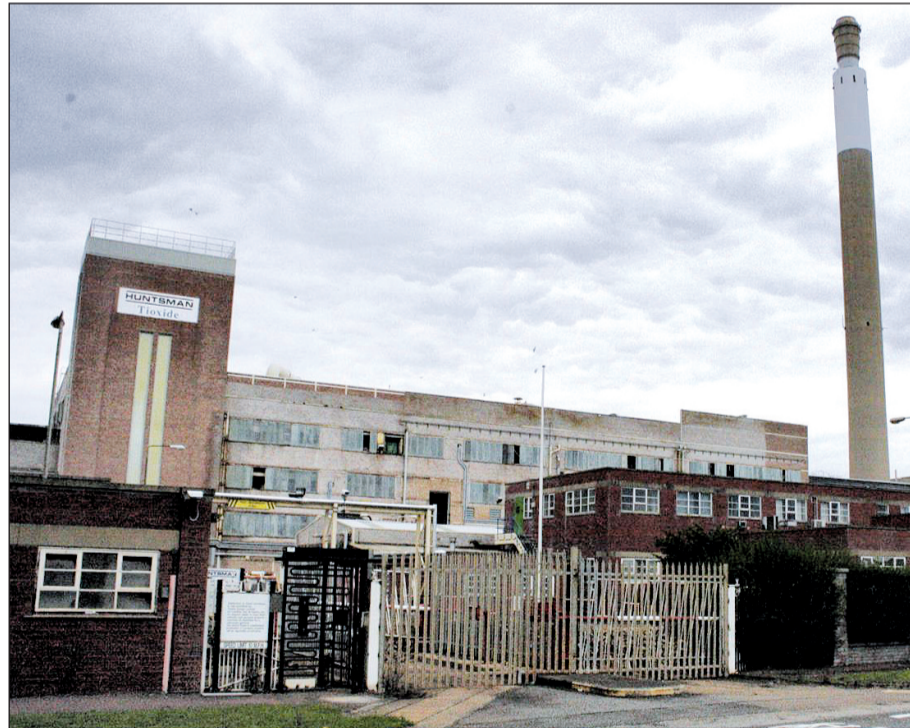
A Grimsby area landmark for many years, the site will soon be cleared.
